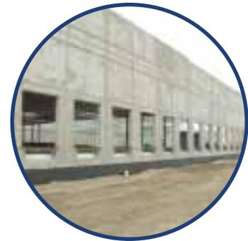
THERMOMASS® insulated concrete panels are load bearing elements. These panels eliminate the need for perimeter structural steel framing and protective curbing. Instead the insulation, structure and cladding are provided in one assembly. Load bearing panels offer significant design and construction savings by simplifying the building perimeter structural conditions. Thus, freeing up interior space for product movement and storage.
