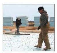
The concrete around the connectors should then be consolidated. Walking on the insulation near each row of connectors and applying foot pressure on each side of the connector can do this effectively. This will cause the still fluid concrete to flow into the notch in the bottom side of the connector.
