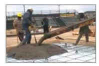
The top layer of concrete is then poured after necessary reinforcement has been placed. This will become the inner (structural) layer of concrete for the finished panel.
